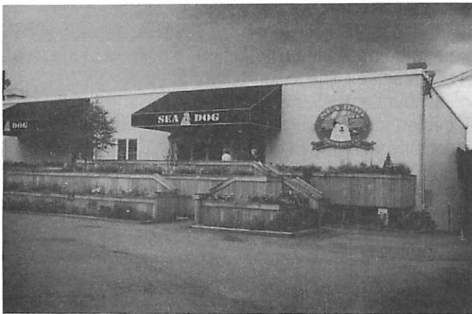
IRP funds were used for this tavern and brewery, when such funds were not to be used for such purposes. OIG photo.
