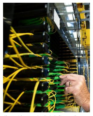
Figure 14. A worker installs fiber optic cables at a data center. Cloud-based computing offers virtualized computing and networking services including off-site data back-up, hosted servers, disaster recovery, and secure data storage. Photo by Lance Cheung from USDA's Flickr account. It does not depict any particular audit or investigation.
