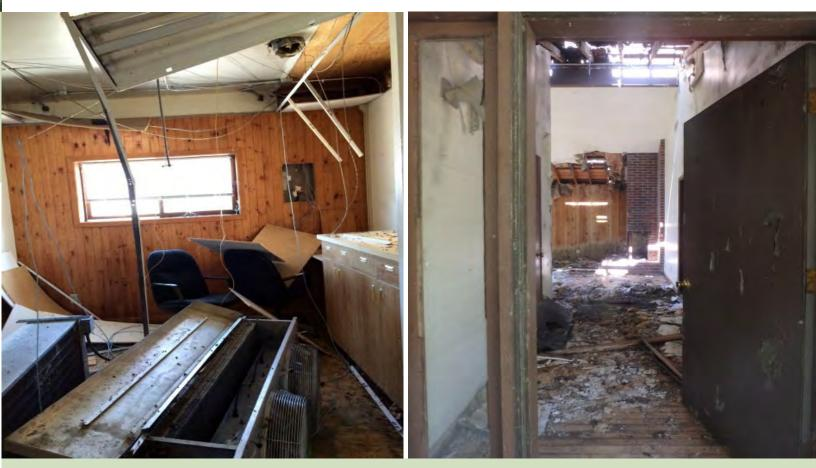
During fieldwork, OIG found buildings with deferred maintenance that had structural issues, mold growth, and widespread rodent droppings.
