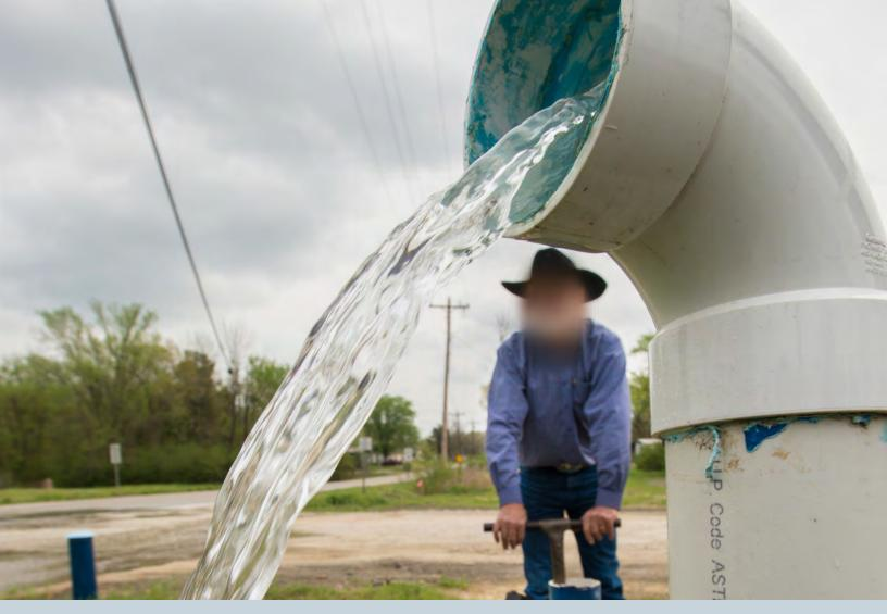
Rural Development provides assistance, such as loans, to help rural communities address water and waste issues. Here, a valve is opened to vent a pipeline, ensuring it is full and properly supplying the community with water.
