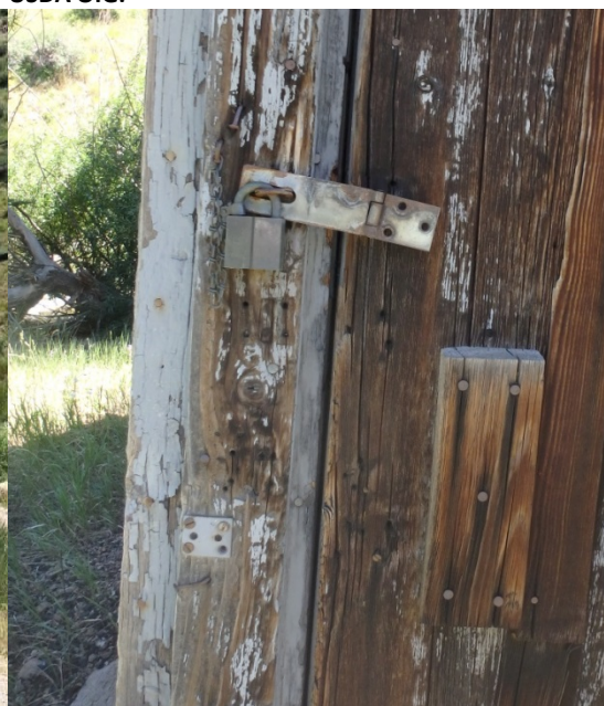
Figure 5: This “red tagged” equipment shed (also shown in Figure 4) was neither secured nor physically red tagged when we arrived on site. A padlock was visible on the latch, but the latch was no longer attached to the door. A section of siding large enough to permit entry was missing from the shed. Photo by USDA OIG.
