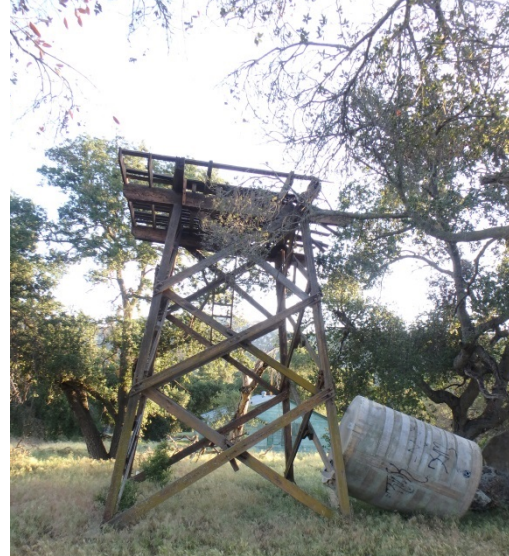
Figure 7: OIG observed a water tower tank that had fallen from its aged wood support structure and evidence of vandalism at the site referred to as “abandoned.” Photo by USDA OIG.
