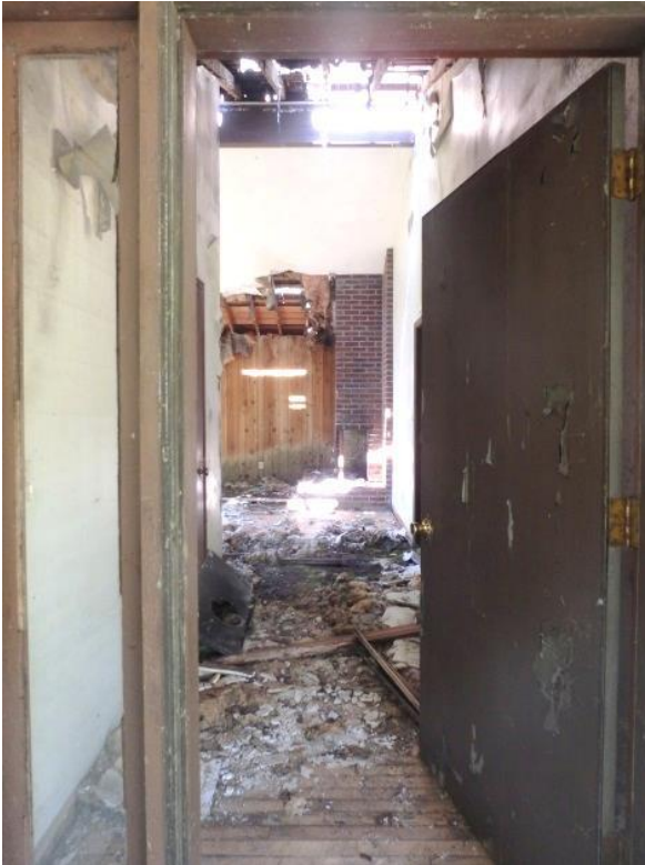
Figure 8: This “red tagged” residential building has a 15-foot wide hole in the roof, fire and water damage, and visible mold across the ceiling and walls. It neighbored other FS residential buildings. Photo by USDA OIG.
