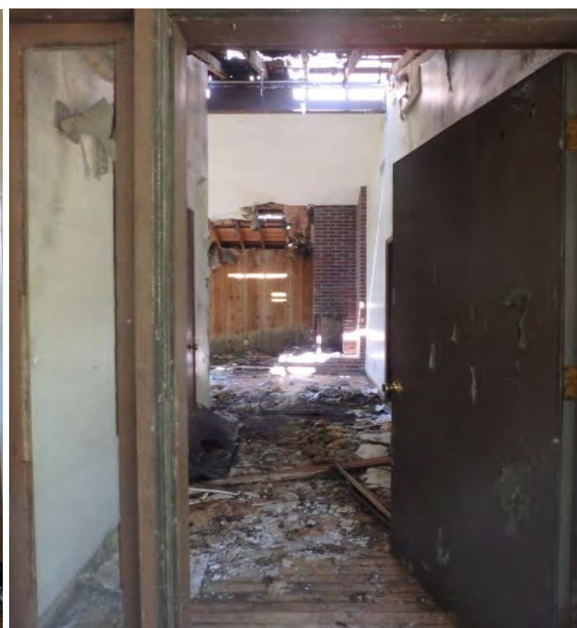
During fieldwork, OIG found buildings with deferred maintenance that had structural issues, mold growth, and widespread rodent droppings.
