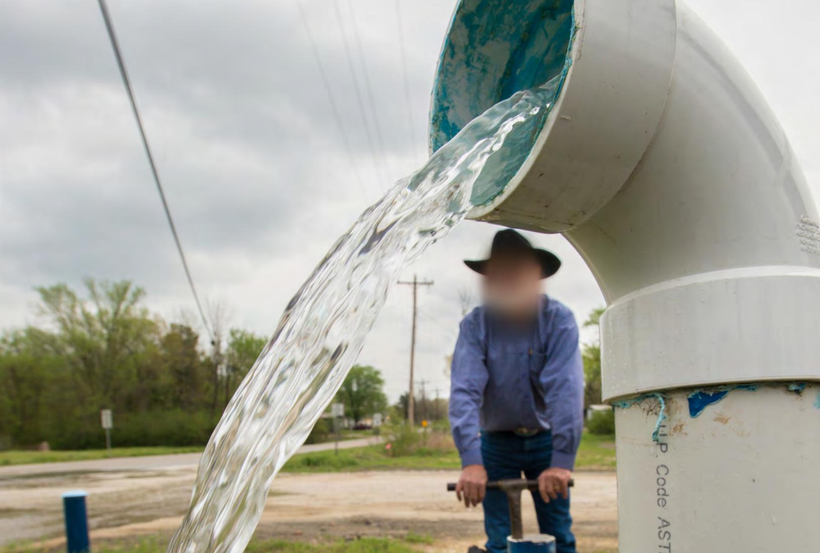
Rural Development provides assistance, such as loans, to help rural communities address water and waste issues. Here, a valve is opened to vent a pipeline, ensuring it is full and properly supplying the community with water.
